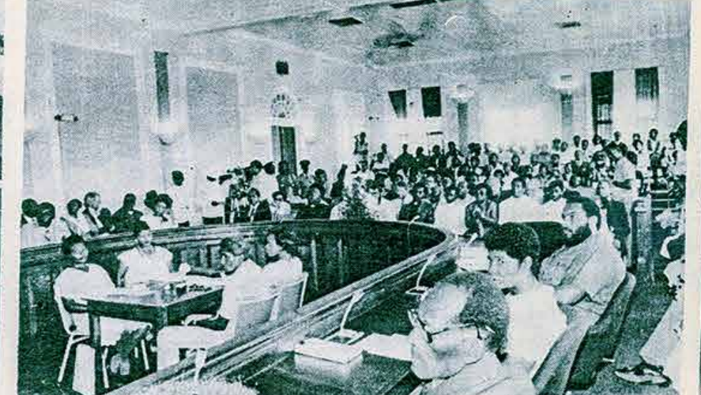
MEMBERS of the Tobago House of Assembly in their newly renovated Chamber.
